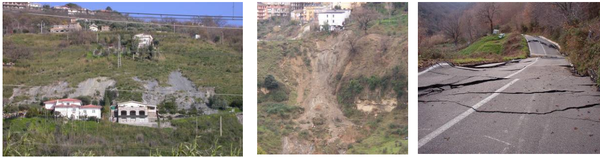
Figure 2. Some effects of the Autumn-Winter 2008/2009 in Calabria. a) top-left: soil slips affecting buildings at Cetraro (CS). b) top-center: earth-fall threatening a building at Petilia Policastro (KR). c) top-right: large earth slide affecting the provincial road at Piano dei Rossi – San Benedetto Ullano (CS); d) bottom left (courtesy of: Maurizio Giglio – Emmegi Arts): the eastern portion of the Cemetery of Fagnano Castello, destroyed by a rotational slide. As a whole, most of the induced landslides were superficial (of either rock/earth fall or earth slide types) which affected many roads and the railway networks, the lifelines and lots of cultivated fields.
