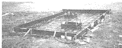
Figure 1. The completed Slab
