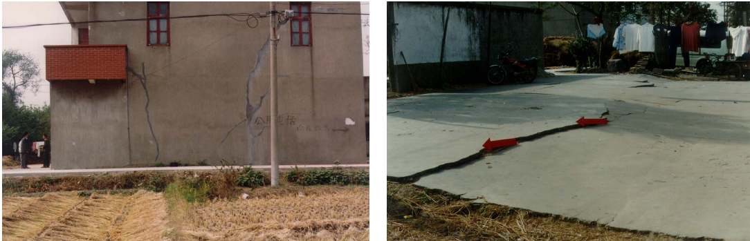
Figure 1. Yinguoan earth fissure, Shitangwan Town, Wuxi City
